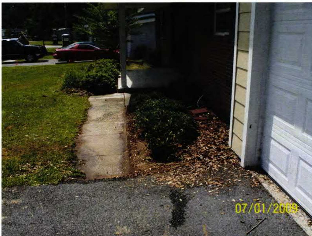
Picture 2: UST 512Laurelbay location after removal of the tank.
